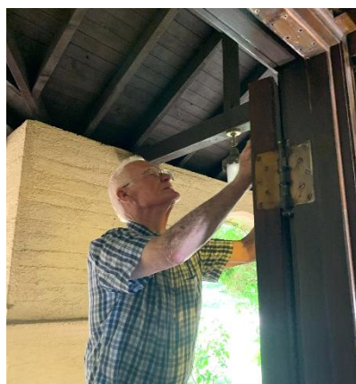
Chris Donnelly installed motorized ADA feature for doors in chapel area
