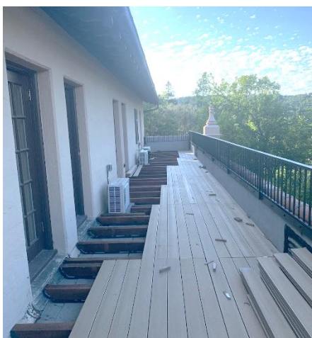
The new deck on the novitiate balcony is under construction; new HVAC units visible
